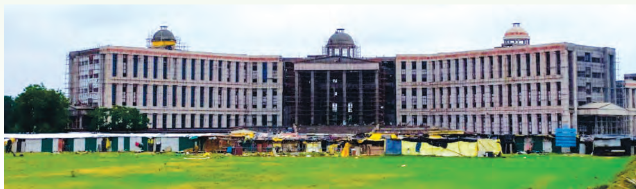
Academic Block under construction
